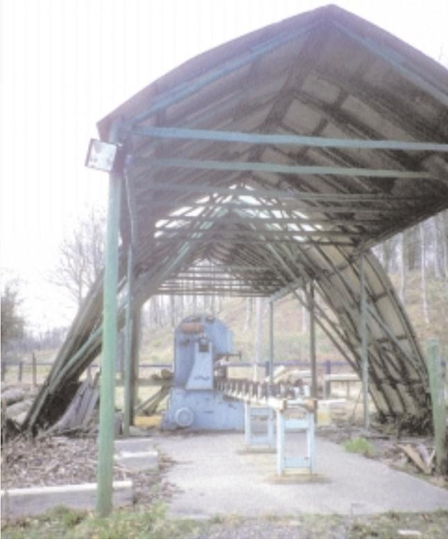
The simple structure shielding the circular saw at Hooke Park. Designed by students from the furniture school, it uses the material agenda of green roundwood with intelligent simple joints to make a small, exemplary, useful building.
